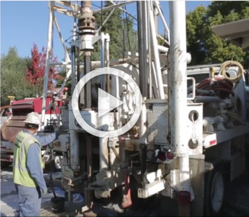
Ground Heat Exchange retrofit installation project in San Ramon, California
